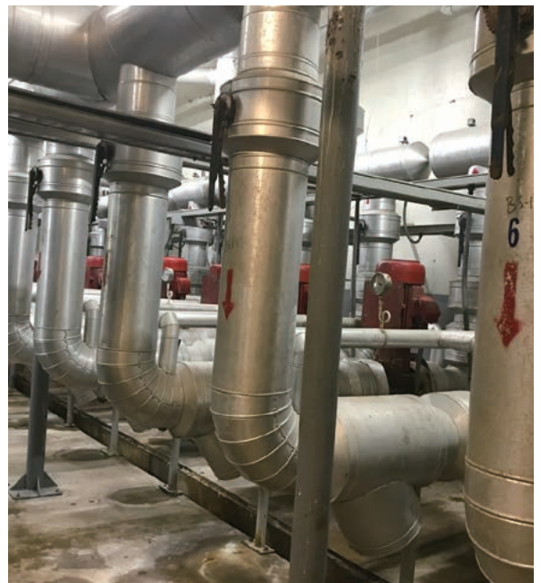
Water pipes and pumps installed in the mechanical room located below the unit.
